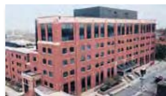
The Christ Hospital Medical Office Building
